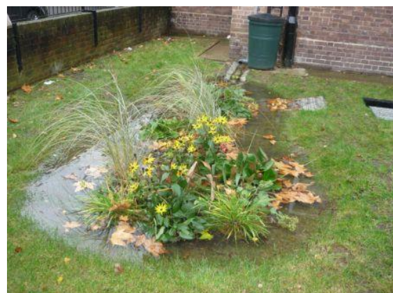
Unlined rain garden close to building foundations (deliberately filled for research)
