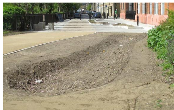
Figure 3 Swale formed, Derbyshire Street pocket park, Bethnal Green, London (courtesy of London Borough of Tower Hamlets)
