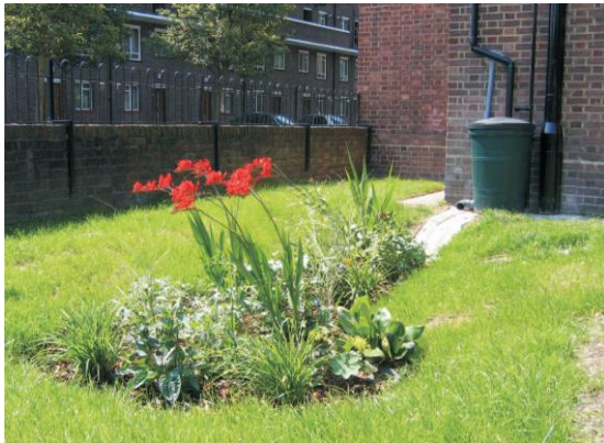
Figure 3 Ashby Grove retrofit rain garden
