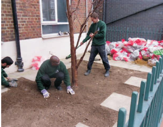
Figure 5 Local residents helping with the retrofit work
