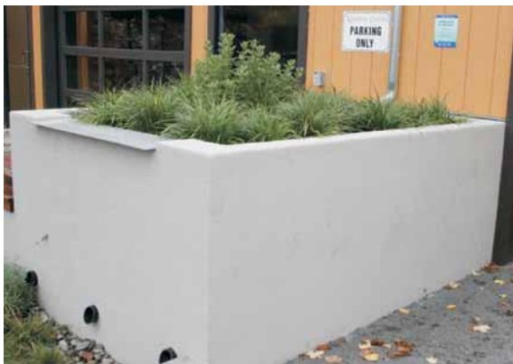
Figure 4 A disconnection planter serving a commercial property (note outreach plaque on the wall) (courtesy DS 7 Photography)
