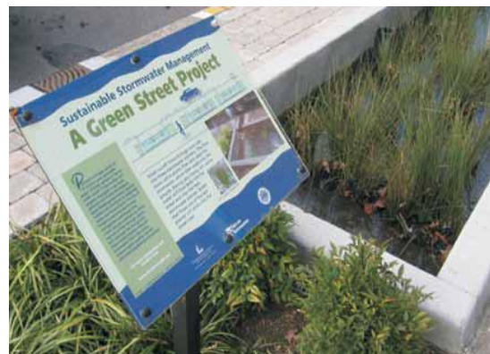
Figure 9 A definitive Portland Green street planter, with informative signboard (courtesy DS7 Photography)
