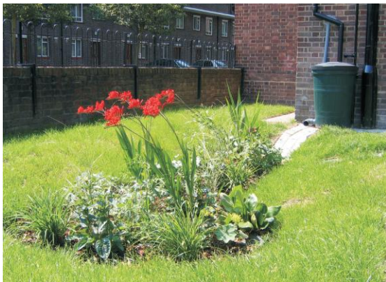
Figure 2 Rain garden situated on a local authority housing estate
