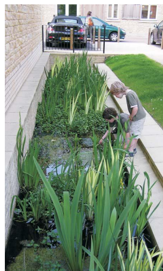
Figure 5 Surface water being effectively managed on a redevelopment site in Stamford (courtesy B Bray)
