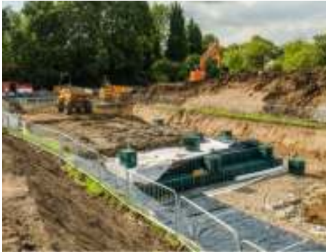
• Herne Hill & Dulwich Flood Alleviation Scheme in partnership with LB Southwark
