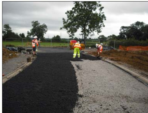
Hand laying 1 st layer of Base
