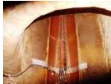
Flow monitor installation for FM512, Lansdowne Rd during low flow conditions
