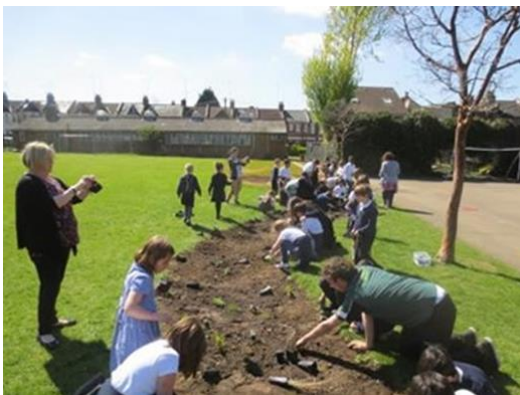
Retrofit SuDS going in at Hollickwood Primary School
