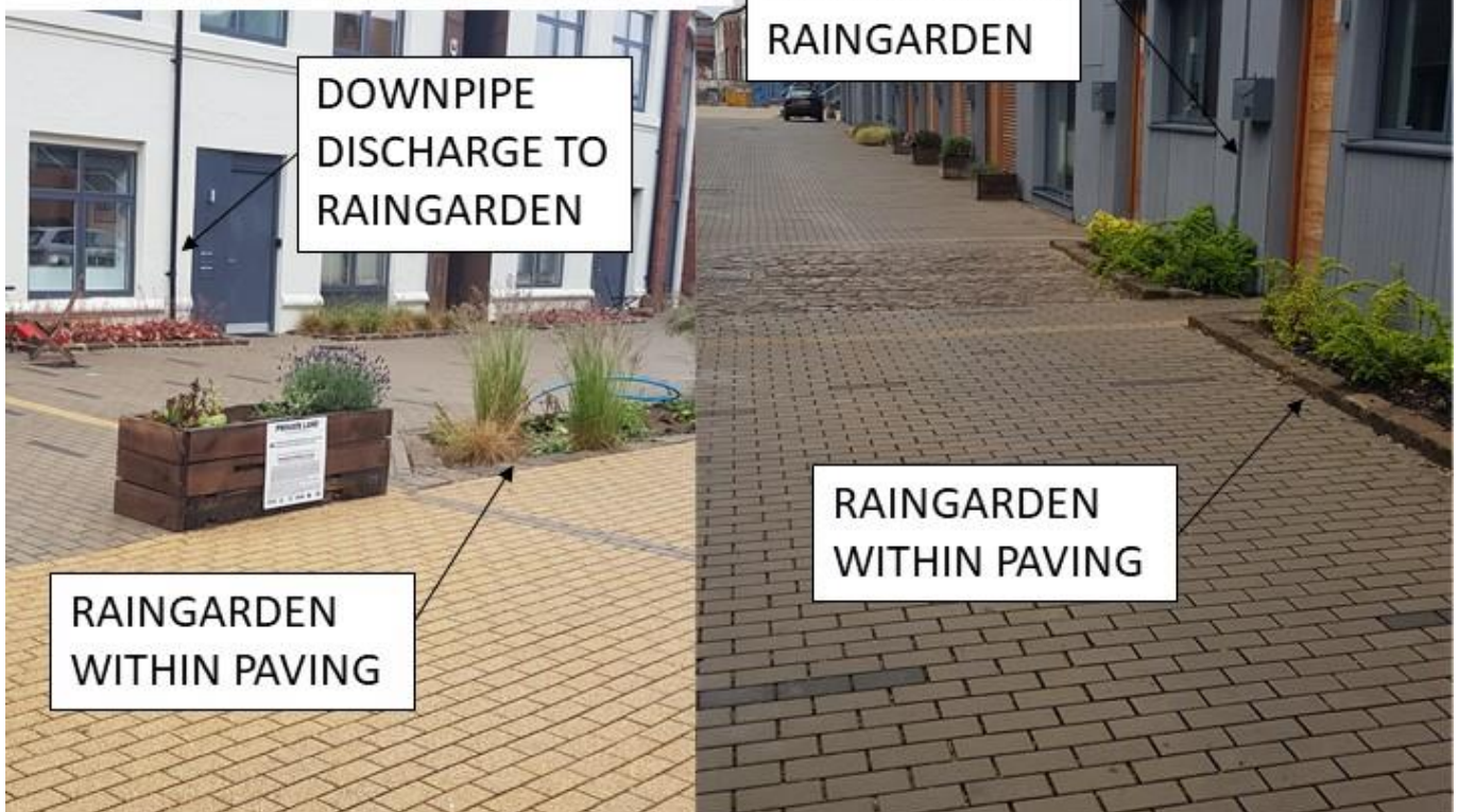
TYPICAL RAIN GARDEN DETAIL WITHIN PAVING PLANTING AND GROWING MEDIUM TO LANDSCAPE ARCHITECTS SPECIFICATION
