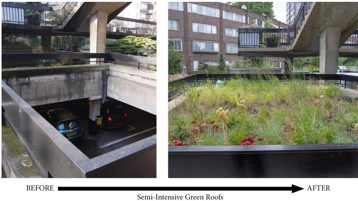
**Fig 4. Semi intensive green roofs over old and polluting car park voids.**
