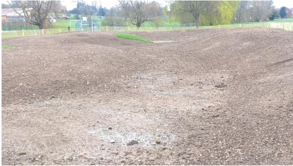
Figure 2: Swale during construction phase – unseeded
