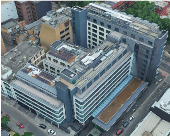
160 Old Street building & roof levels
