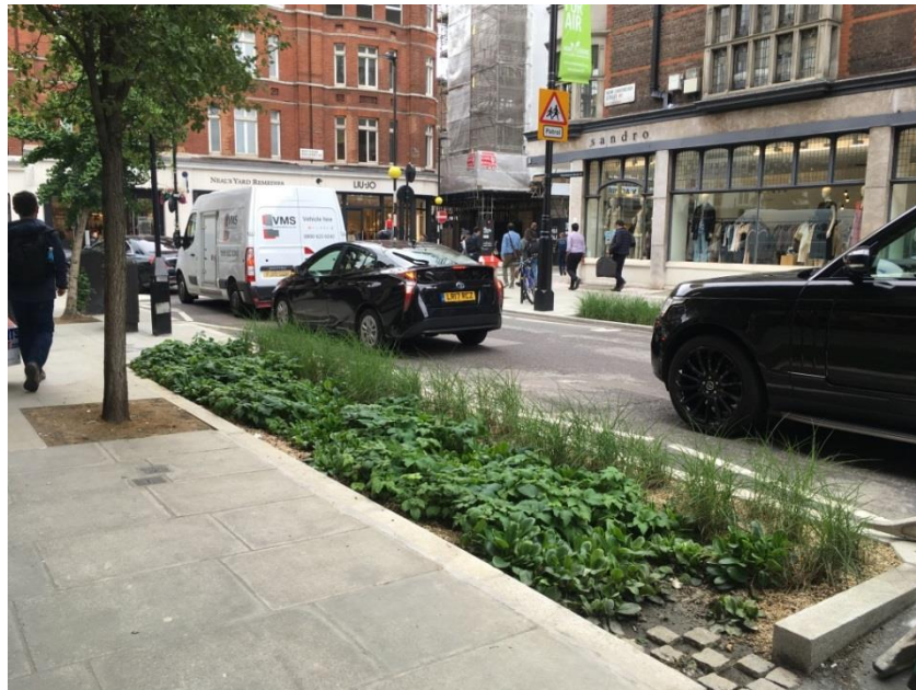
Image 1: Rain Gardens in Package 6 – View west towards Marylebone High Street (Aug 2019)
