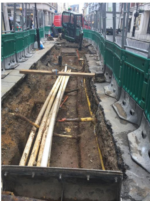
Image 4: Rain Garden Package 3.3 – Existing utilities and below ground structures (Feb 2019)
