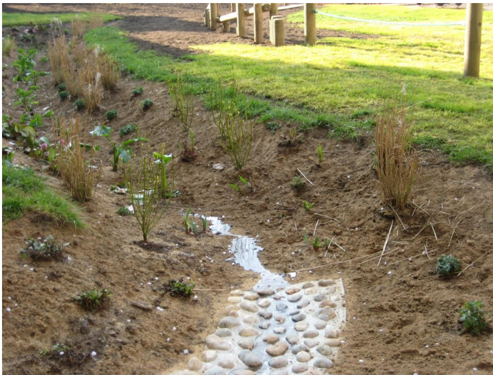
Water discharge into Rain Garden during construction
