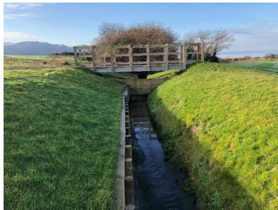
Figure 5 Timber weir and footbridge
