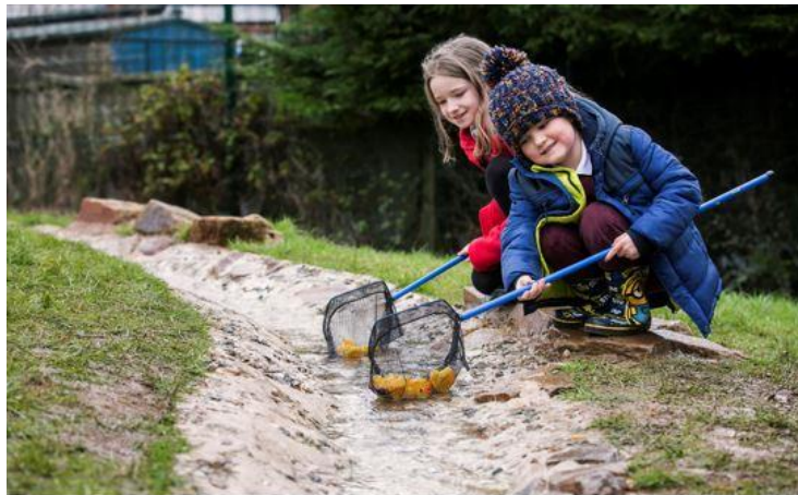
Fig. 2 – The rill transfers flows from the geo-cellular tank to the detention ponds.
