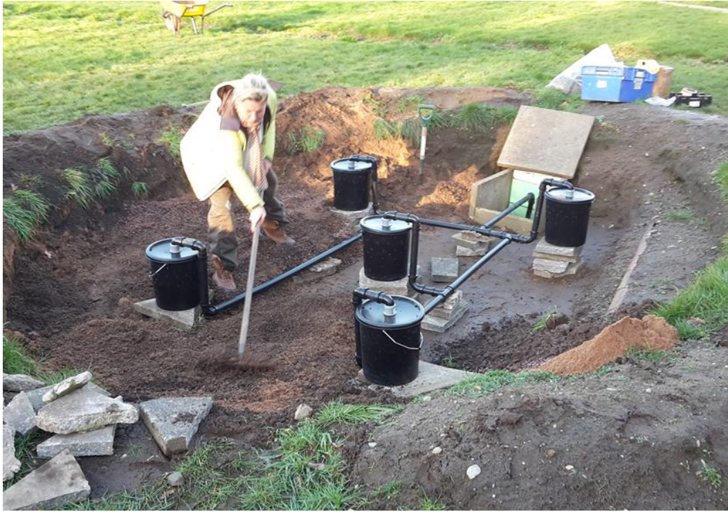
6. Testing silt-trap buckets being for water-flow
