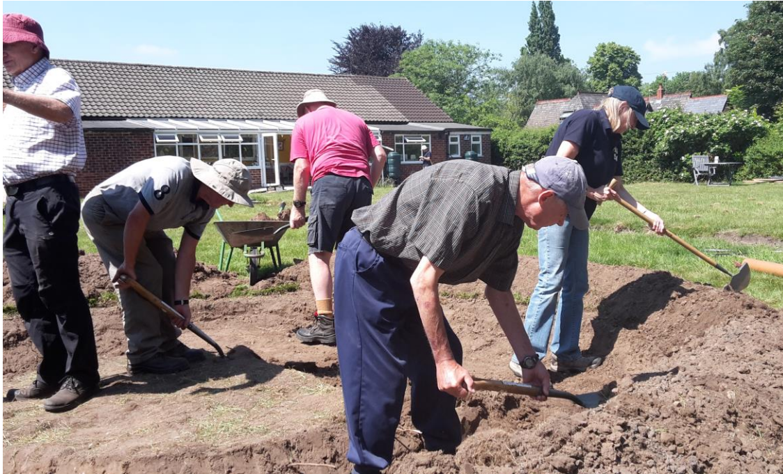
4. Vale Royal Conservation Volunteers excavate the pipe trenches
