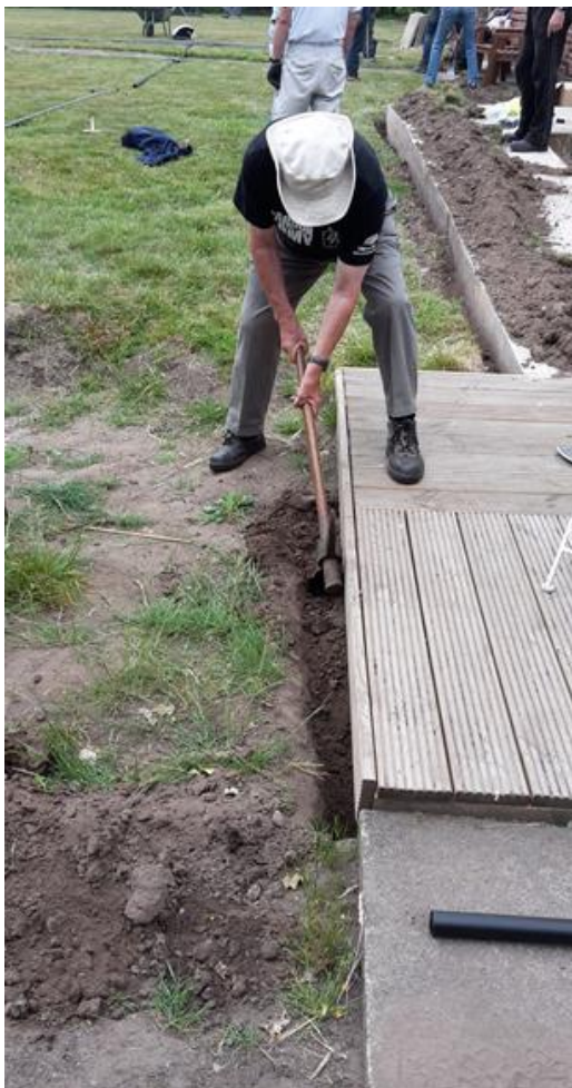
5. Love My River Volunteers installing five-point outfall and silt-trap buckets
