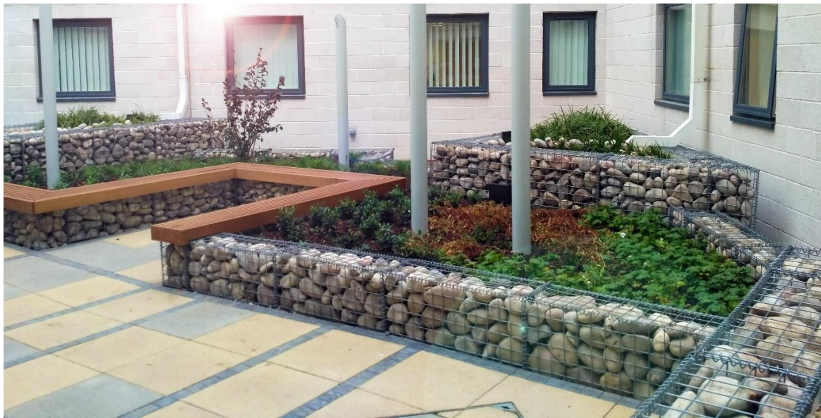
Infiltration and low-level planters in Café Courtyard.
