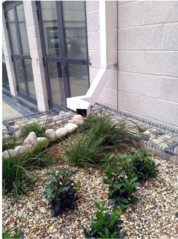
Downpipe diverted into new infiltration planters.
