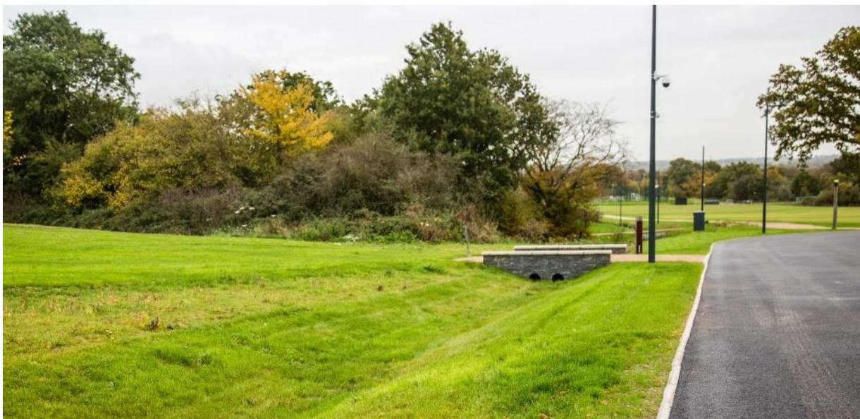
Fig 5 The estate perimeter road drains via sheet runoff across a 2m wide filter strip at 1:20 into a 3m wide swale.
