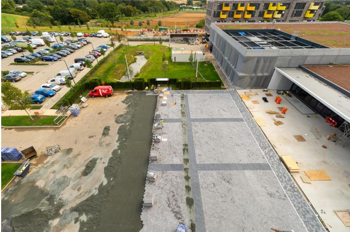
Fig 4 Permeable paving under construction at arrival plaza; discharging to treatment pond behind. Green roof on adjacent reception and service/events buildings.
