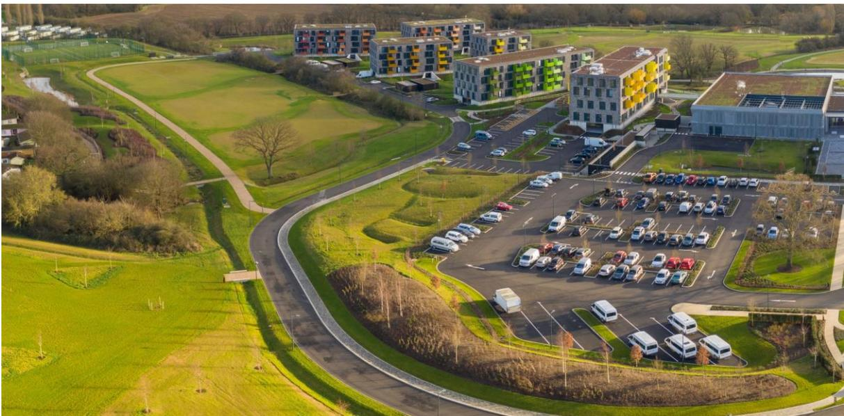
Fig 7 View of east half of development: roadside swale in foreground; porous asphalt parking areas discharging to swales; attenuation pond at back left.
