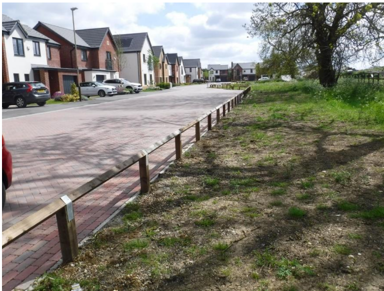
October 2019; showing the drainage at grade into the filter drain
