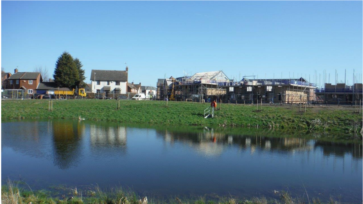
Housing almost complete; landscaping still to happen
