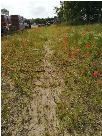
Keeping the swale shallow – house construction stage
