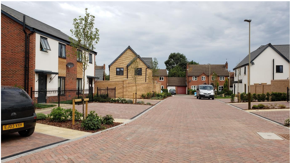
Permeable paving through the 'mews' street summer 2019
