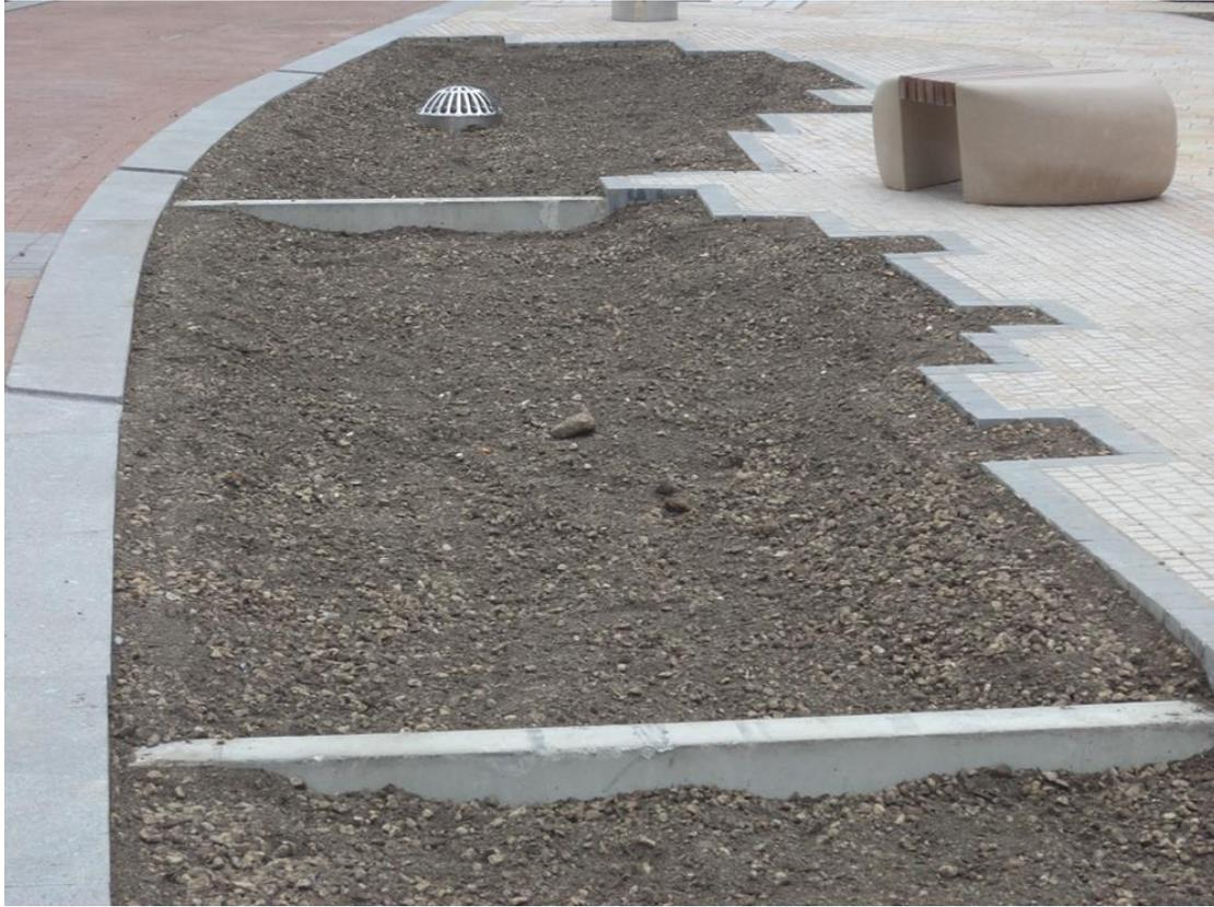
Load bearing lintel surface flow check dams in the Linear Bio-swales pre planting 2018
