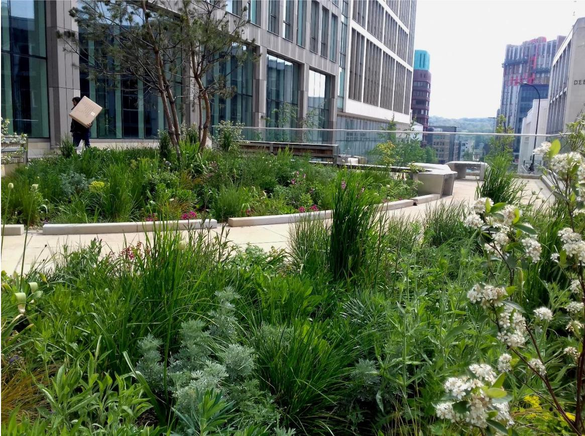
Bio-swales gardens with enhanced storage beneath paving. This is a podium construction with 550mm of total depth including storage beneath. The planting acts as a bio-filtration inlet protecting the storage cells beneath.
