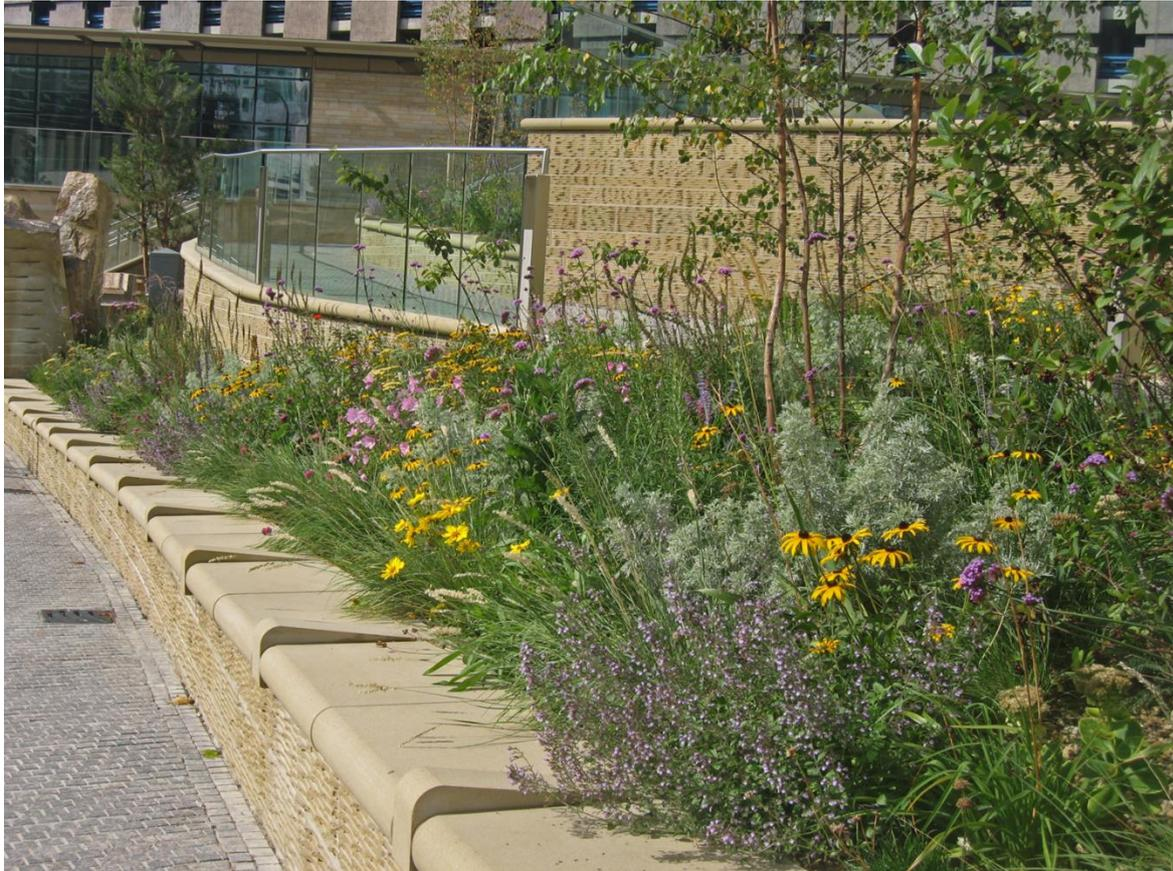
Terraced Bio-retention gardens. 4m of level difference over underground loading bays provides an opportunity to play and enhance the water storage and treatment of surface waters as we collect at higher levels, outfall to lower levels and continue to recollect through infiltration at the lowest areas. These plantings are part of the active water management design of the scheme
