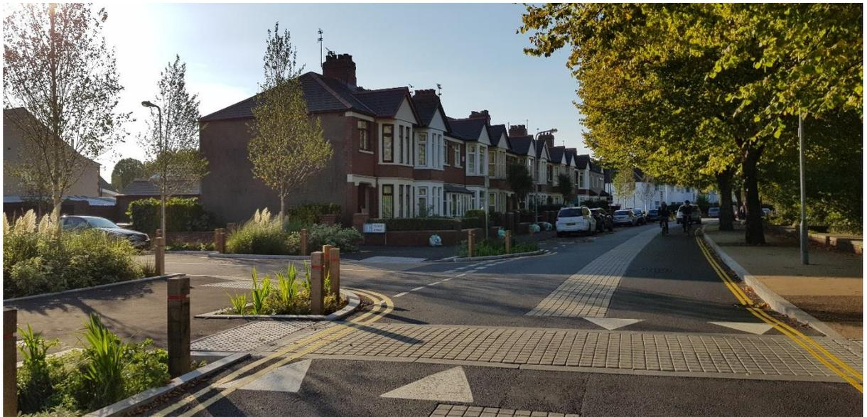
Figure 7 - Bicycle street, safer junction and widened pedestrian footpath along the Taff Trail
