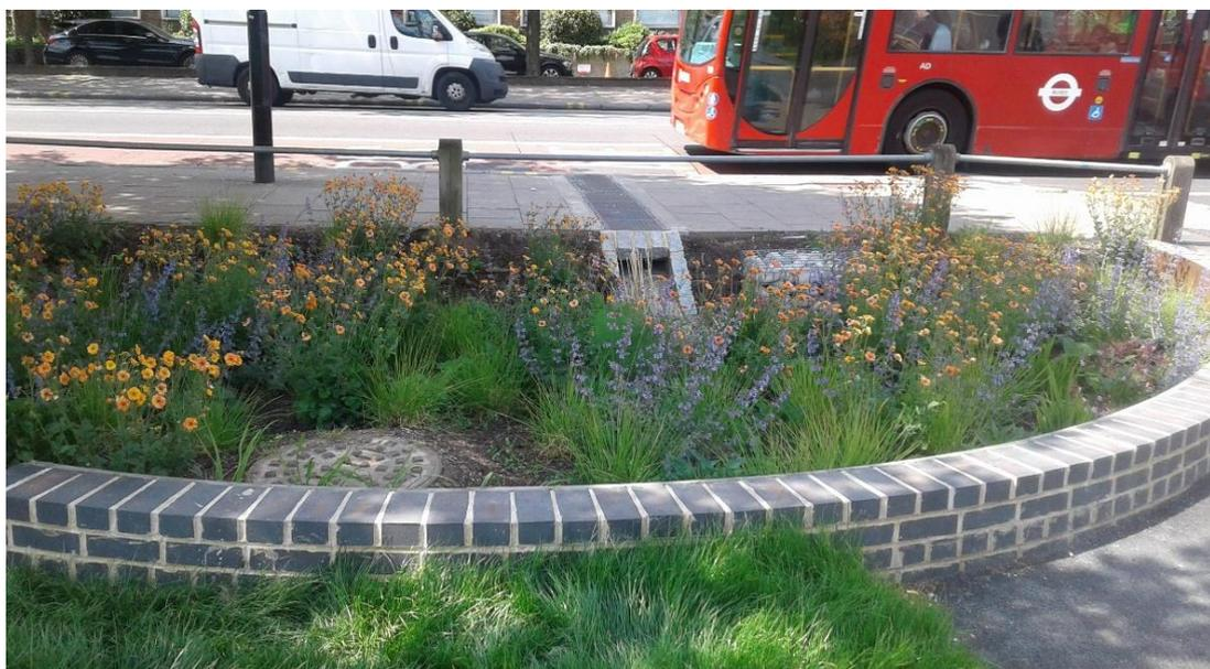
**Fig. 2: Established Rain garden - Collecting surface water during storm event**
