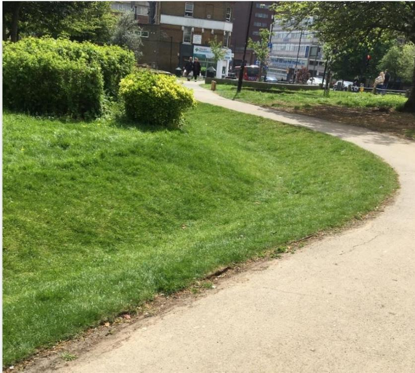
**Fig. 7: Longest Swale within Park connecting rain gardens at both ends**
