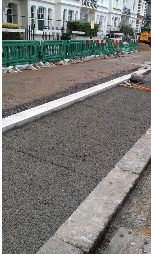
Figure 3: Just laid pervious concrete – Eddiscombe Road
