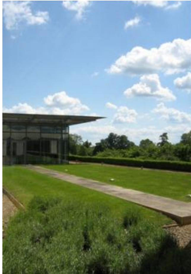
Figure 3 Green roof (Wessex Water)
