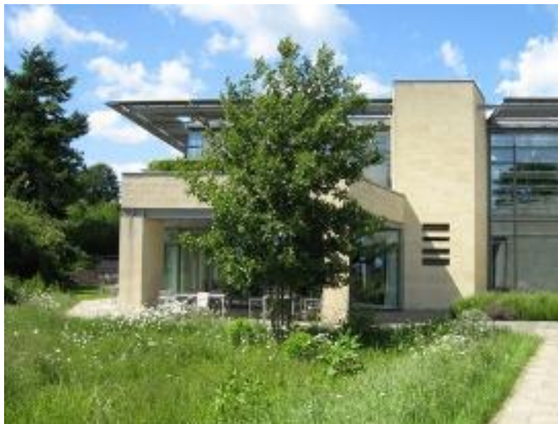
Figure 2 Floodable area (Wessex Water)
