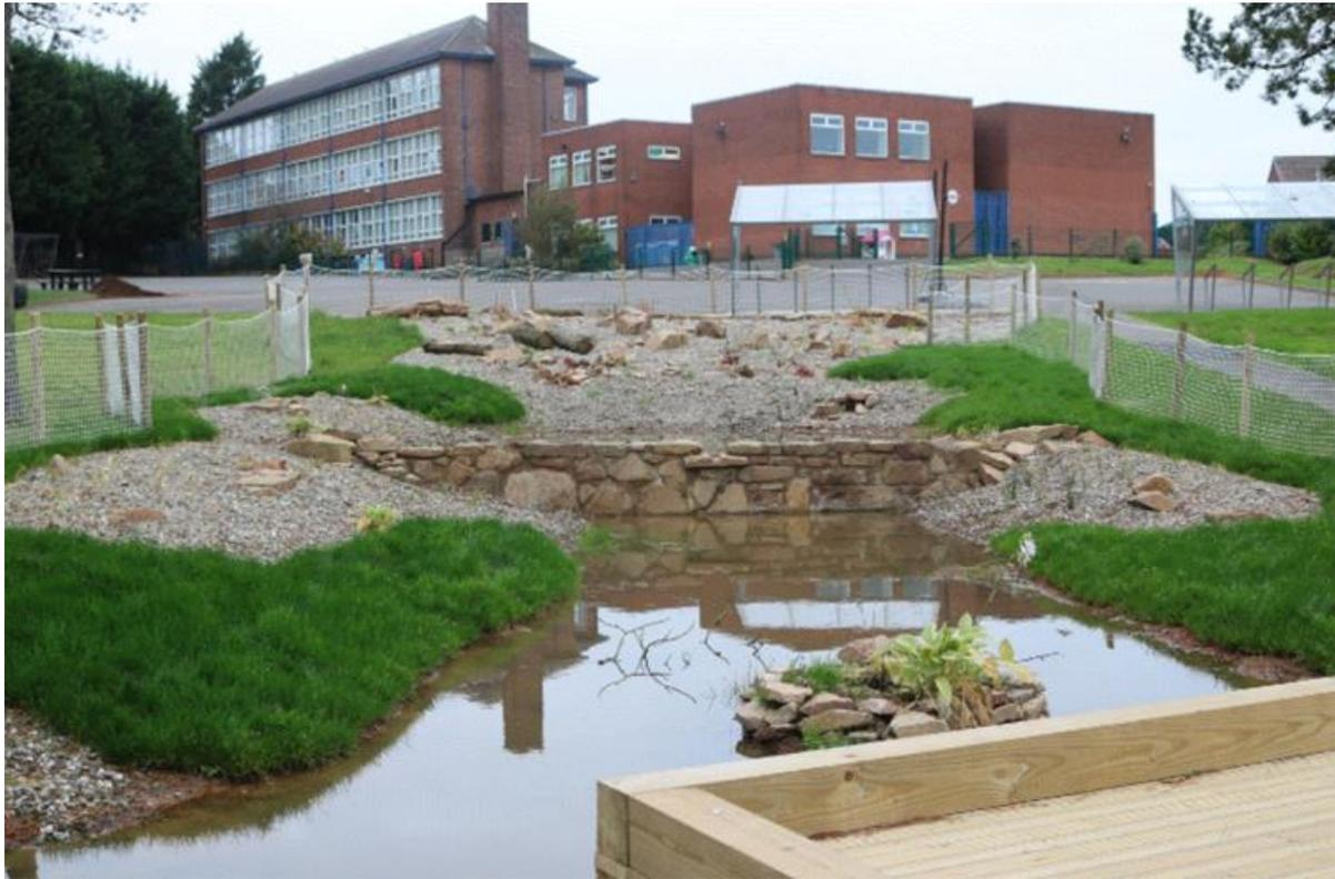
Fig 2: Pond B and weir wall
