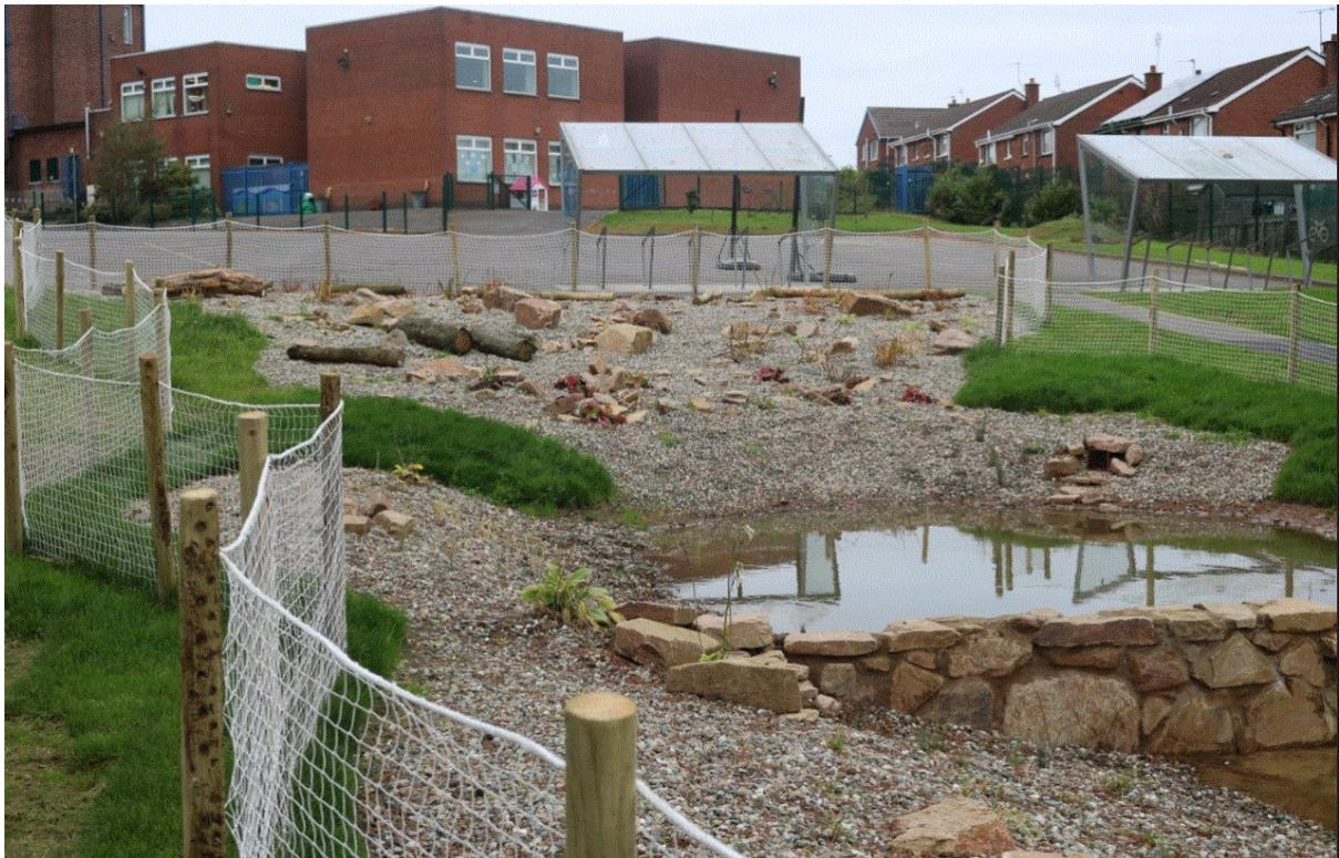
Fig 1: Pond A with Bog Garden collecting hardstanding runoff
