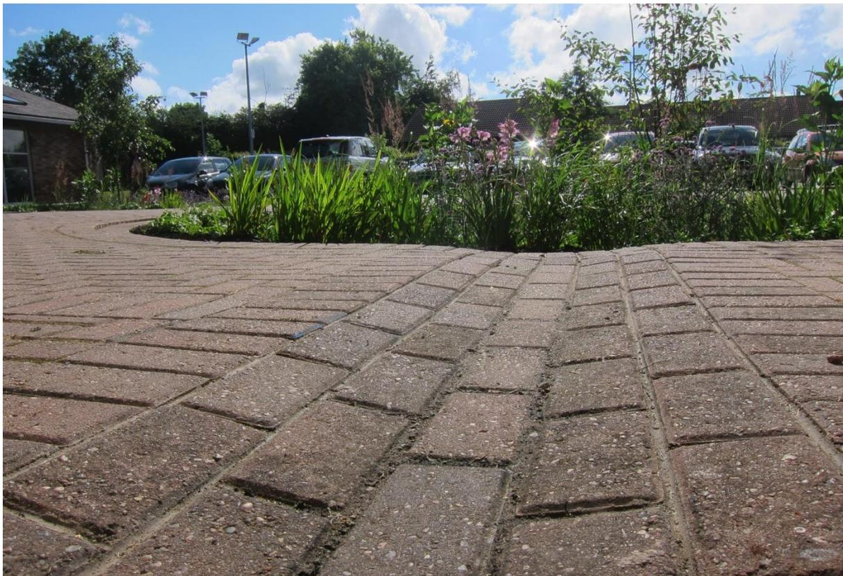
Fig 4: Raingarden Inlet Channel, Year 1
