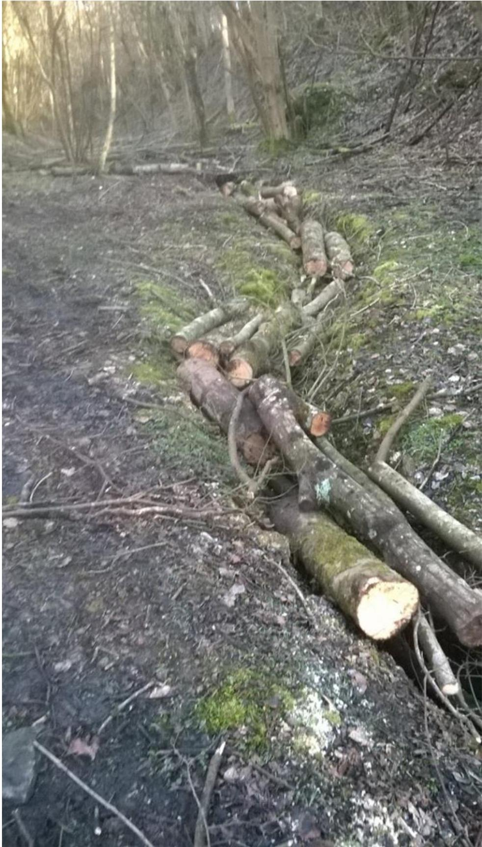
Fig 3: 6<sup>th</sup> Jan 2016 stuffing erosion gullies with wood in the Upper Slad valley
