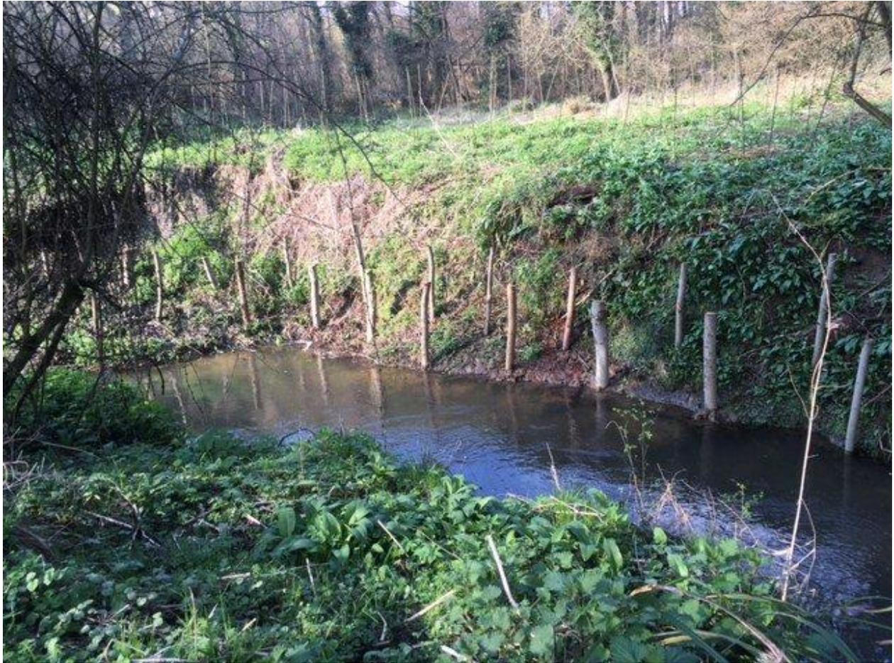
Fig 4: Willow stakes used on the Painswick Stream at Wick Street Farm to help reduce bank erosion.
