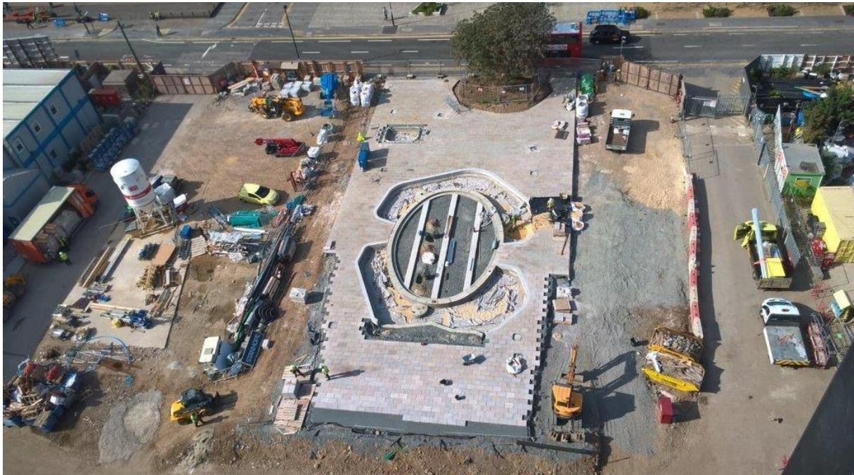
Fig 4 Grit-jointed permeable paving installation, September 2016. © Lendlease
