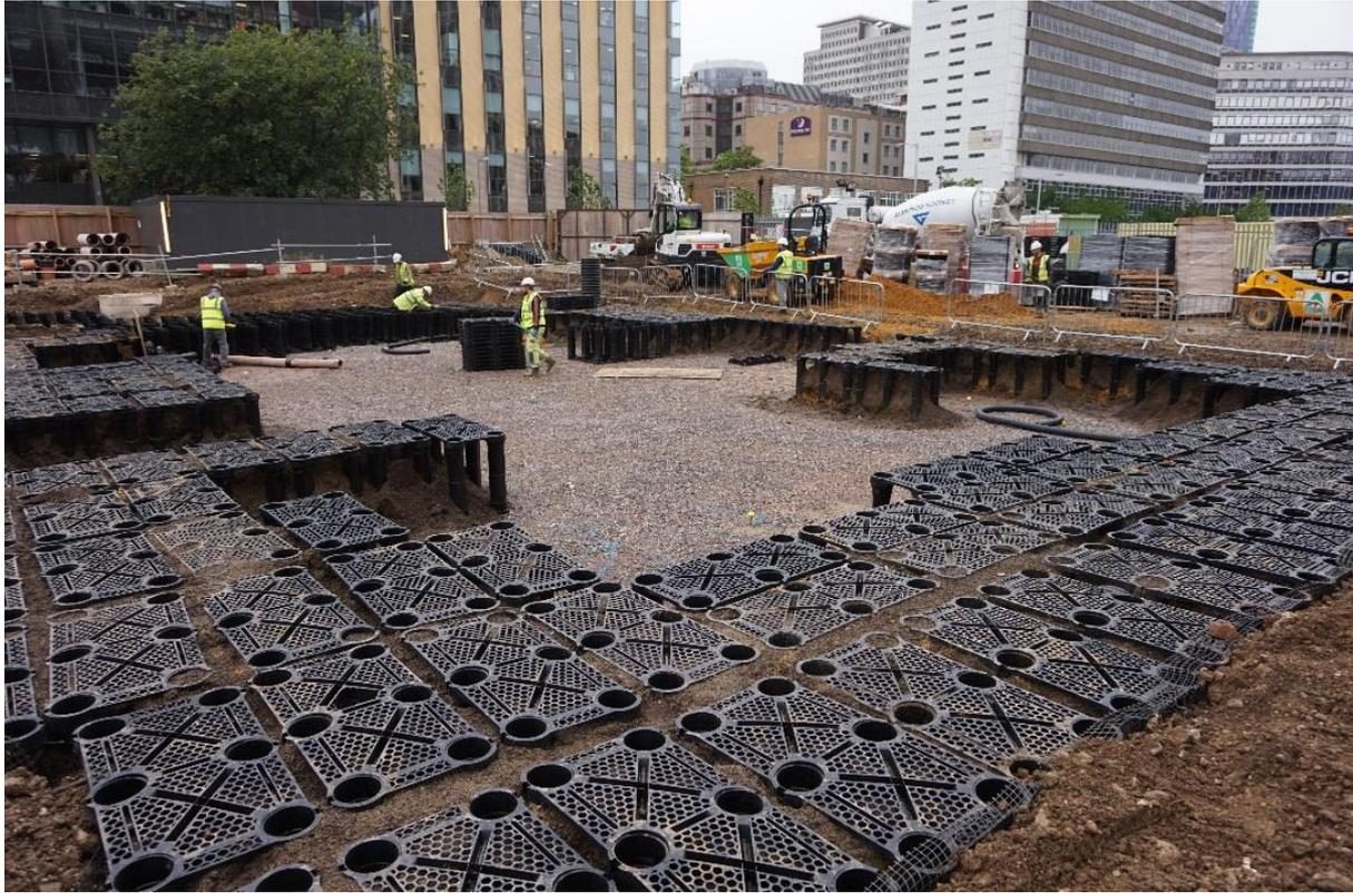
Fig 3: Soil cell installation, June 2016. © J & L Gibbons
