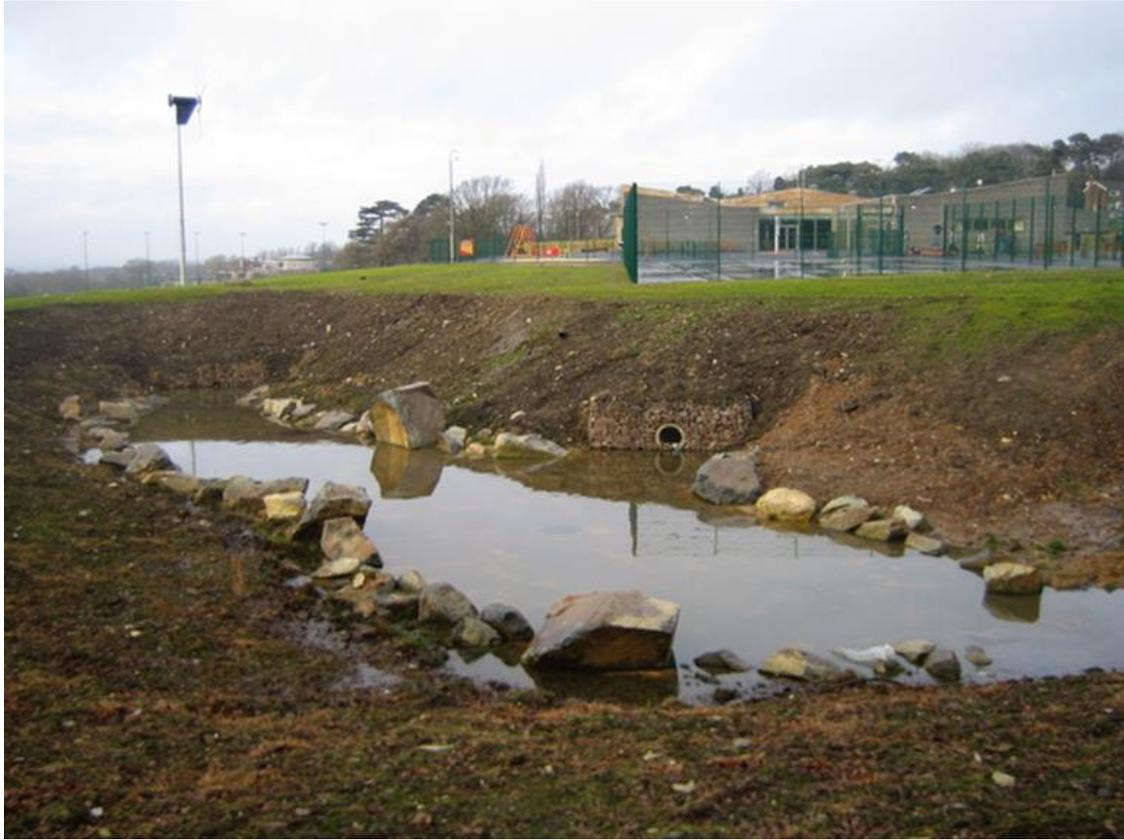
Fig 3: SuDS shortly after construction and un-vegetated
