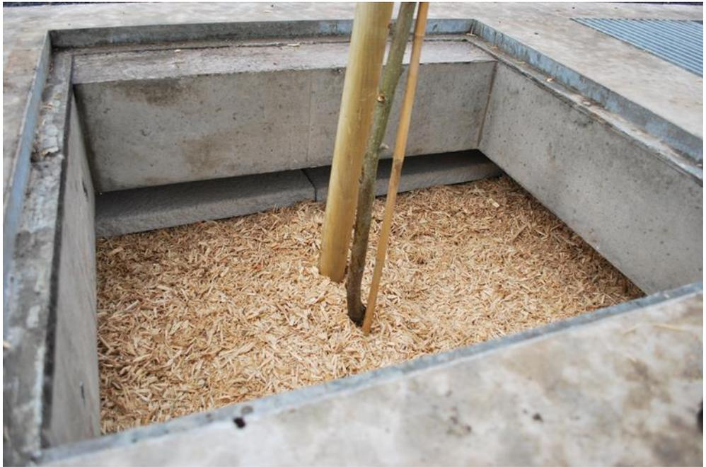
Fig 3: Installation of mulch layer
