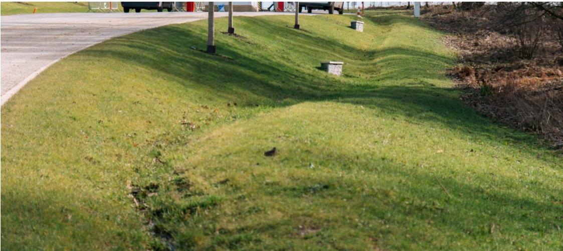
Fig 7 Roadside swale with outlet headwalls
