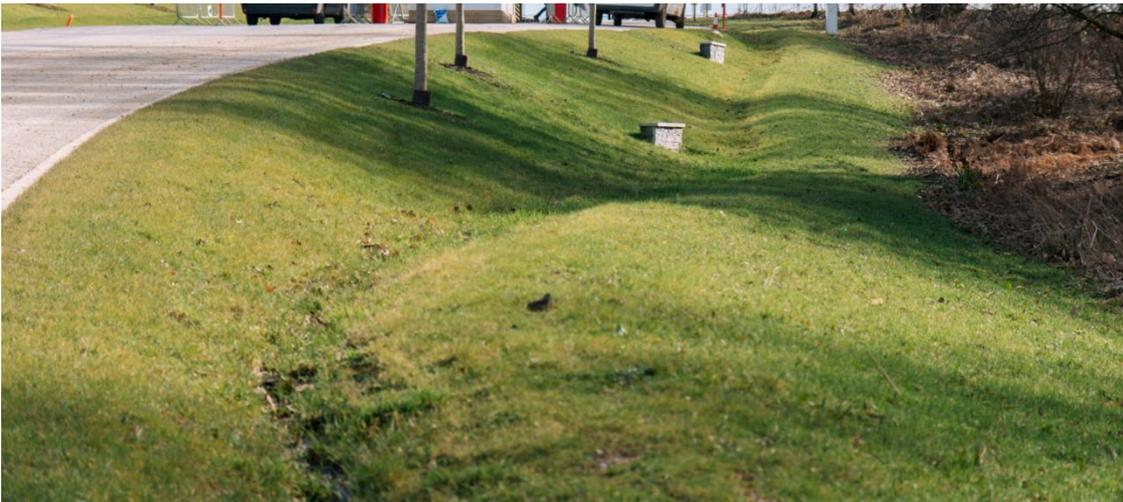
Fig 7 Roadside swale with outlet headwalls
