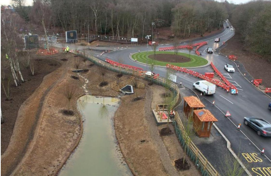
Fig 2 Soft landscaping works underway at the attenuation pond (
