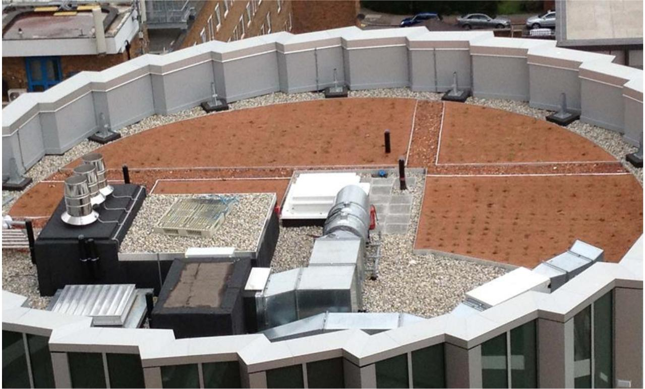
Fig. 8: Mixed finish roof
