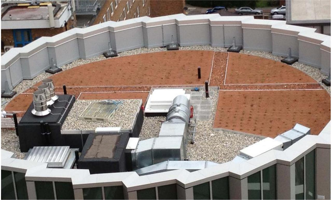
Fig. 8: Mixed finish roof
