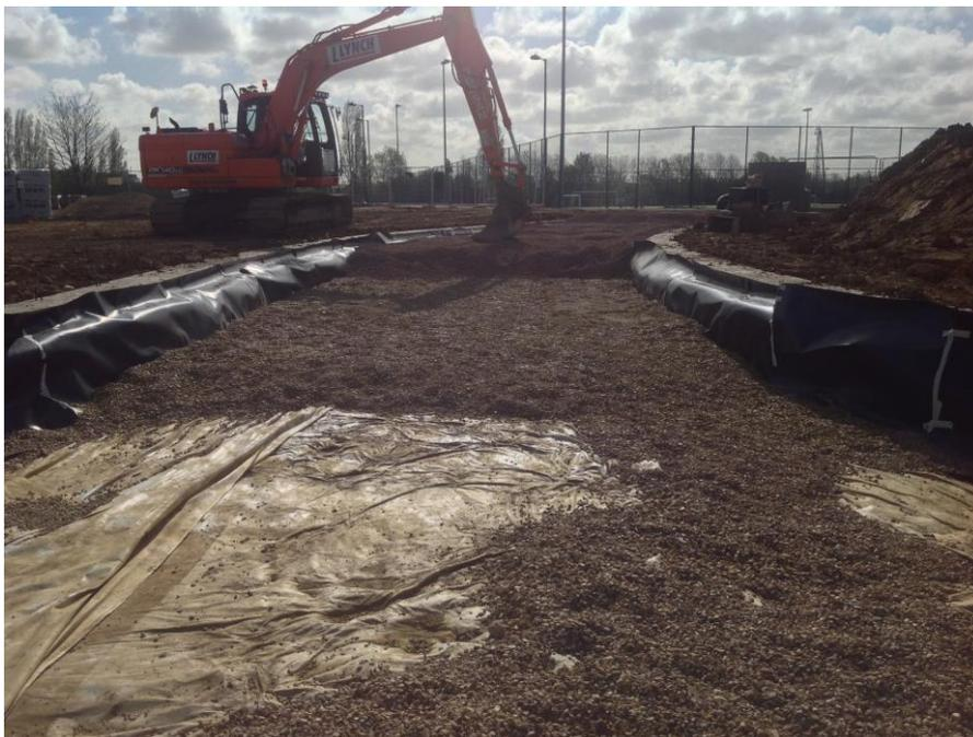
Fig 3: Laying of permeable sub-base
