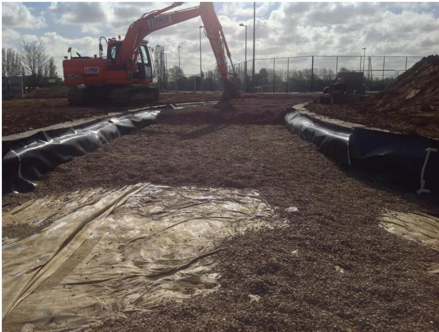
Fig 3: Laying of permeable sub-base
