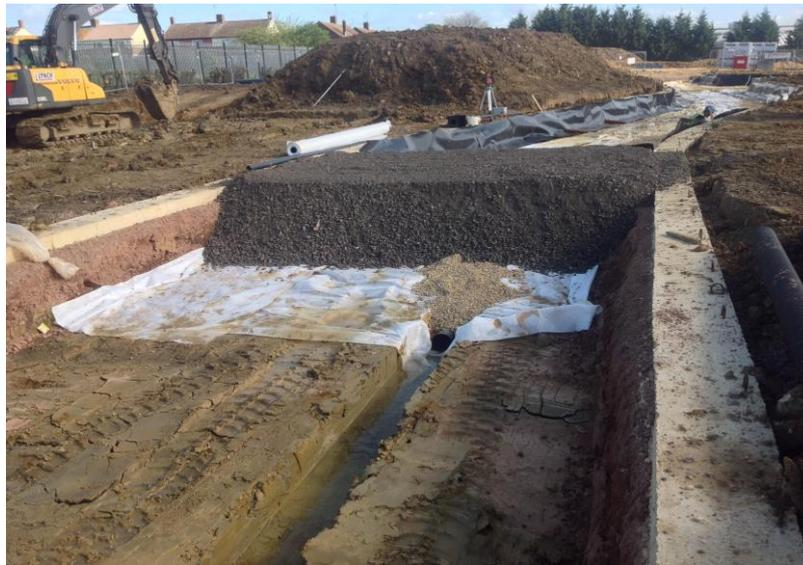
Fig 1: Impermeable service corridor
