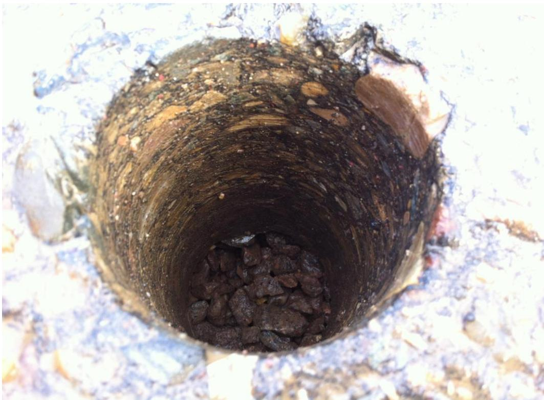
Fig 5: DBM core showing permeable sub-base beneath
