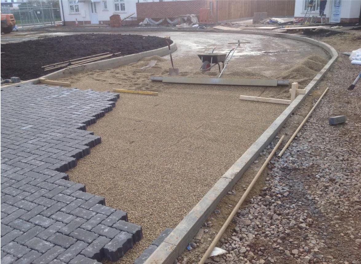
Fig 6: Laying the permeable blocks
