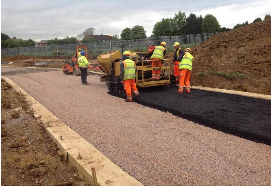
Fig 4: Laying of DBM on permeable sub-base
