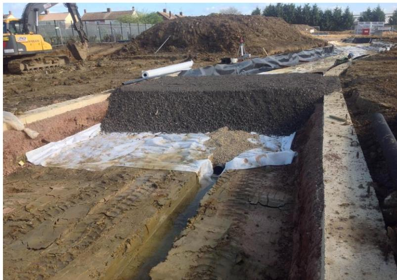
Fig 1: Impermeable service corridor
