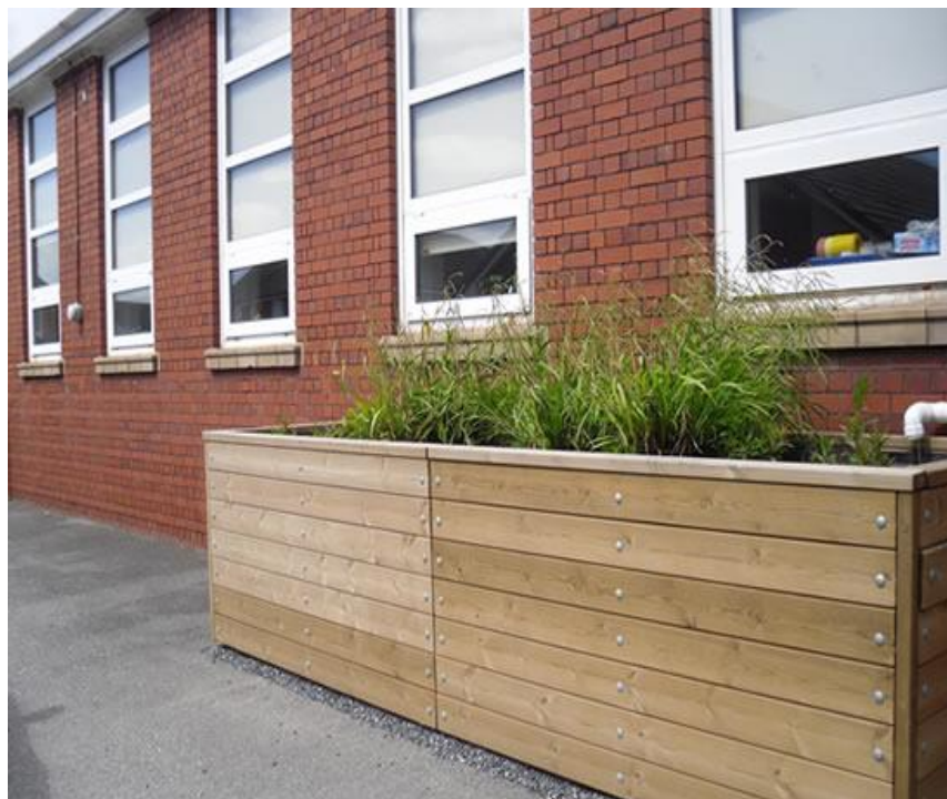
Figure 7 Rain planter on the car park elevation of the school
