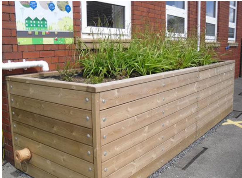
Figure 2 Downpipe disconnection into rain garden planter
