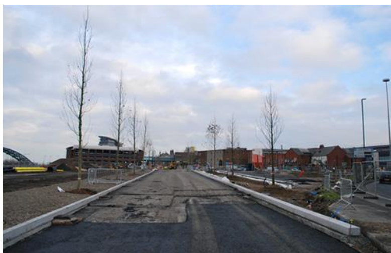
Figure 3 The new road
