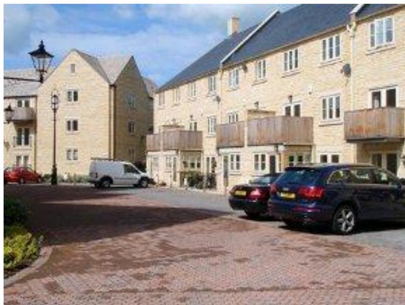
Figure 2 Car park using permeable paving (Bob Bray)
