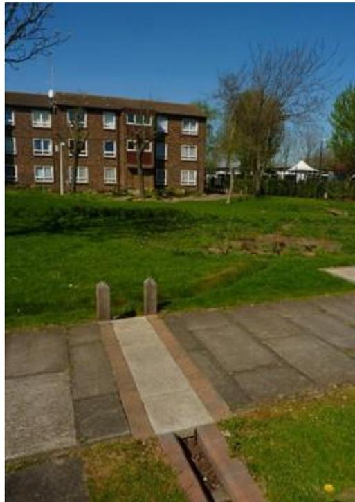
Figure 2 Ornamental rain garden (early after installation) showing a channel bridge under a pathway
