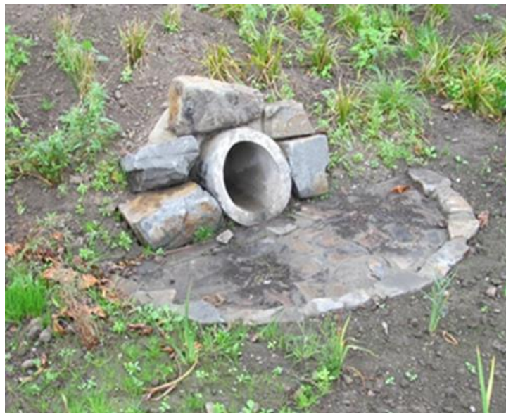
Figure 1 Outfall from highways network into the swale
