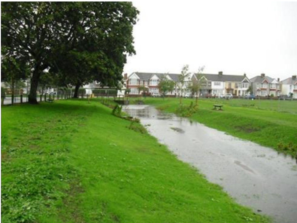
Figure 3 Swale becoming full
