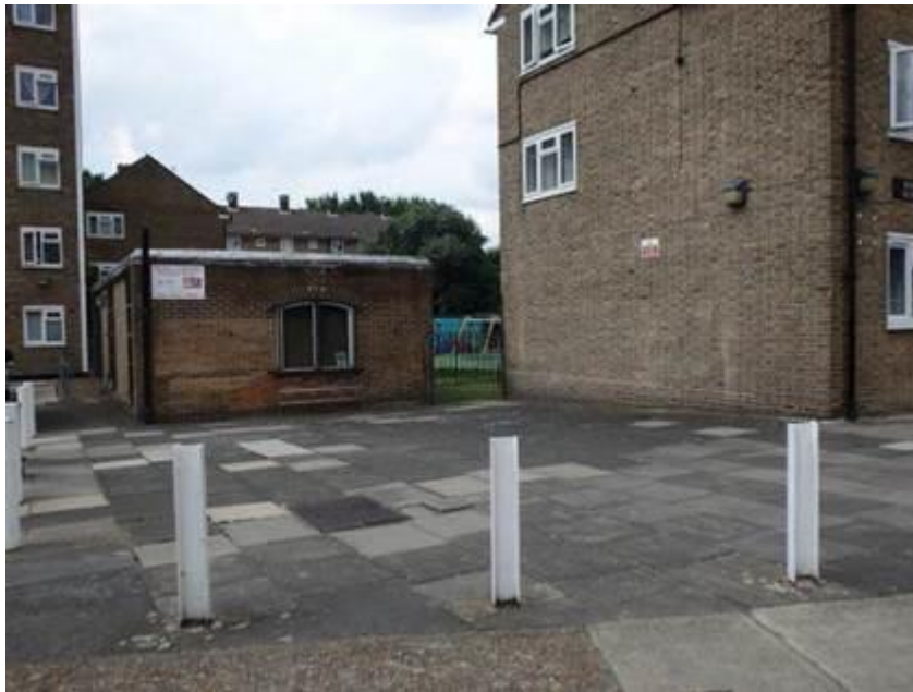
Figure 1 Prior to SuDS construction
