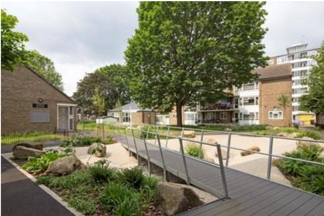
Figure 6 Stony detention basin
