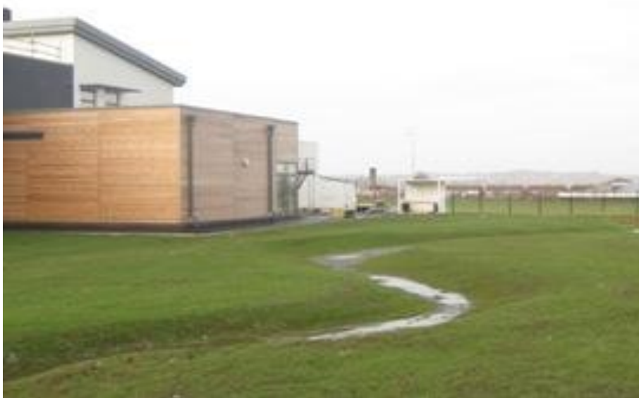
Figure 10 The curvilinear form to the swale system, combined with ground modelling and planting, creates a series of outdoor spaces to be used for teaching (David Singleton)
