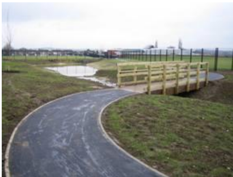
Figure 9 The main detention basin with the new pedestrian bridge installed in January 2011. This allows people contact with the water system, and an elevated view of the basin and sedge shelf (David Singleton)
