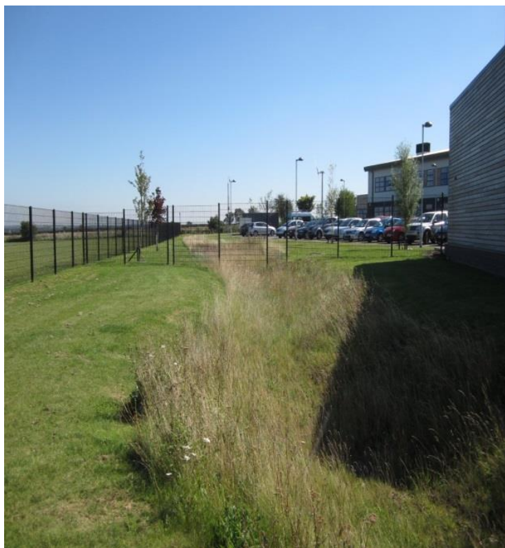
Figure 6 The swale system carries water through a 'nested wetland' to a main dry detention basin
