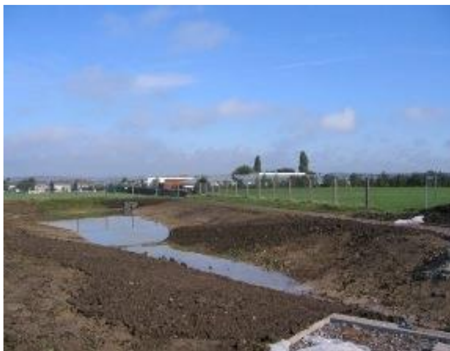
Figure 8 The main detention basin showing the elevated 'sedge shelf' close to the new pedestrian bridge in October 2010 (David Singleton)
