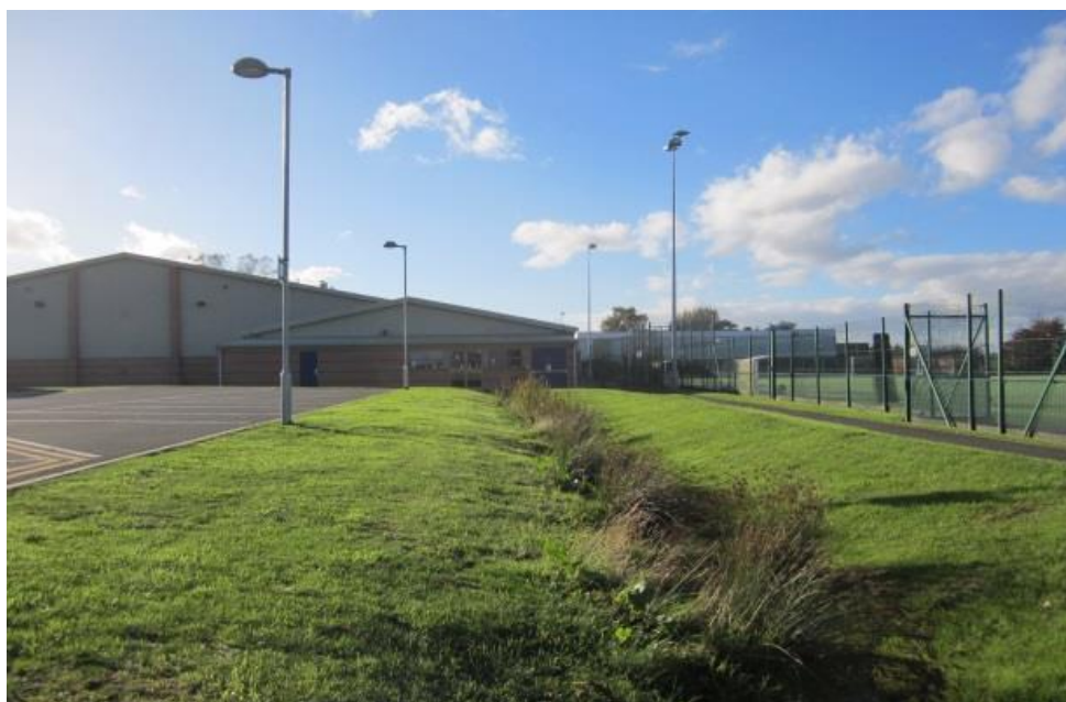
Figure 7 The swales are shallow and have carefully graded slopes to enable mowing
