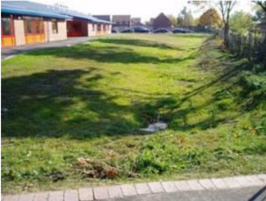
Figure 1 Main drive storage basin with controlled outfall (Bob Bray)
