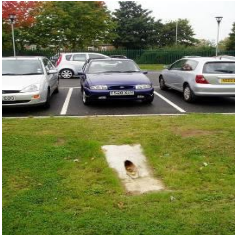
Figure 4 Car park inlet (Bob Bray)
