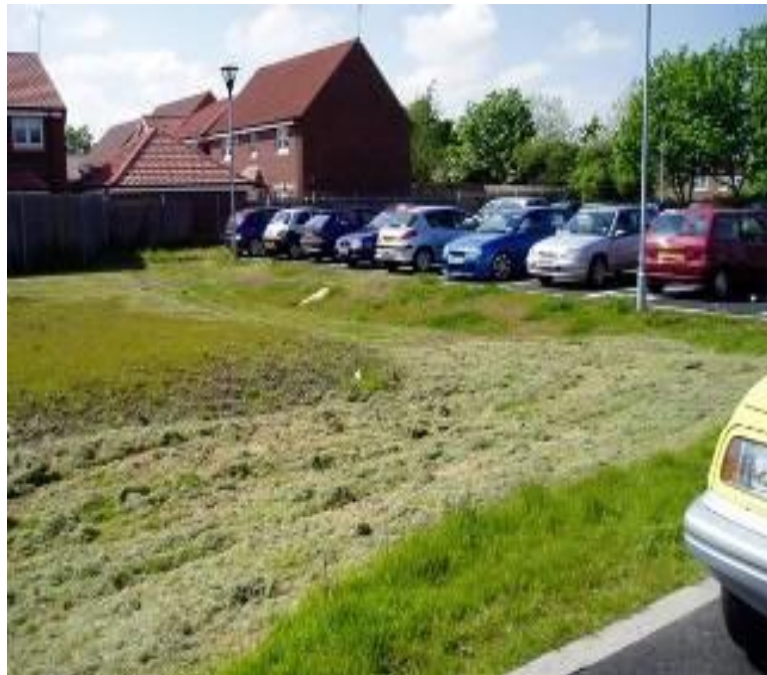
Figure 5 Car park collection swale (Bob Bray)
