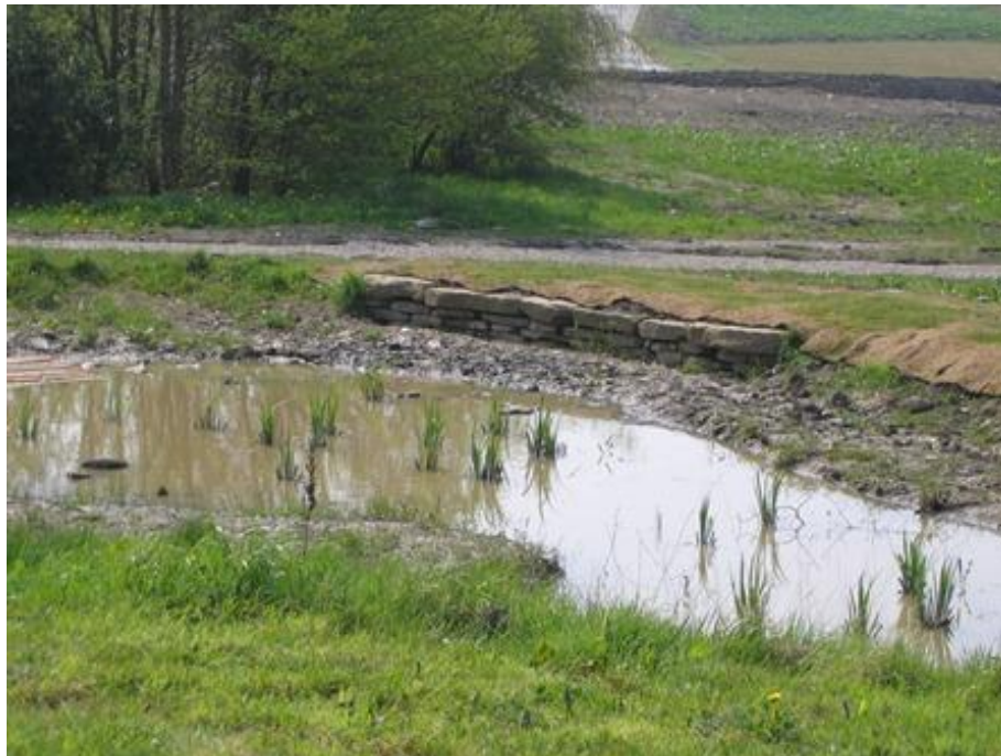
Figure 3 Turfing used to vegetate vulnerable areas of the system (Roger Nowell)
