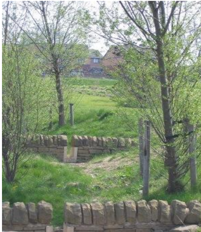
Figure 2 Swales that run through the site with inlet/outlet structure
