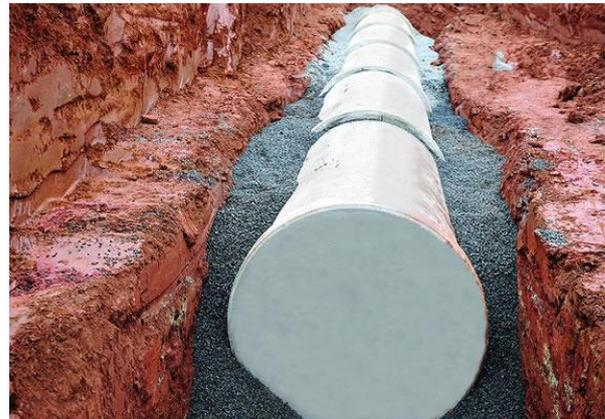
Figure 4 Concrete pipework
