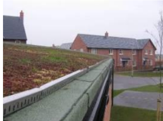
Figure 4 Green roof on bike shed (Royal Haskoning)
