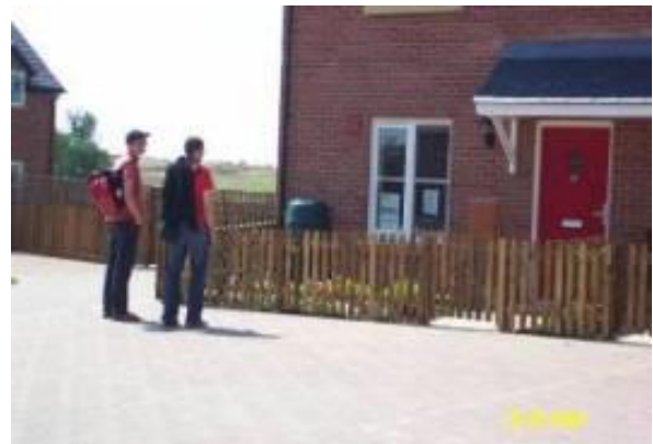
Figure 2 Permeable paving (Royal Haskoning)
