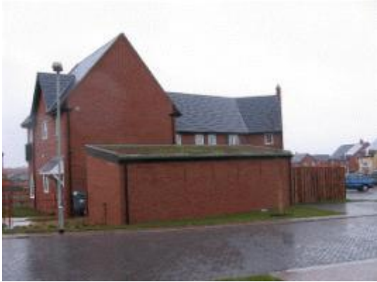
Figure 3 Green roof on bike shed (Royal Haskoning)
