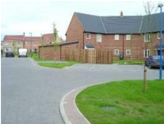
Figure 1 Permeable paving (Royal Haskoning)
