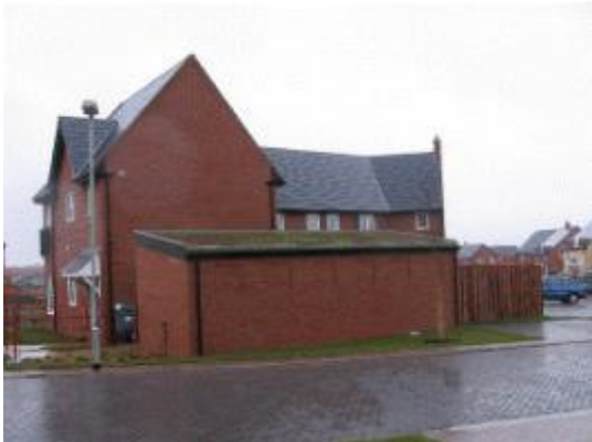
Figure 3 Green roof on bike shed (Royal Haskoning)
