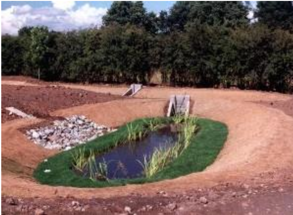
Figure 1 Spillage basin newly constructed (Bob Bray)
