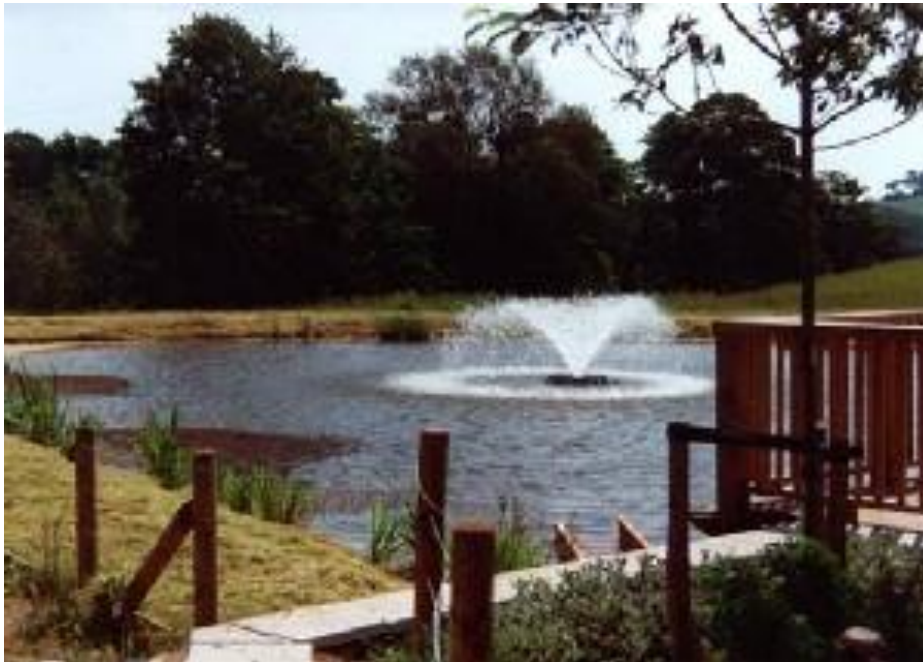
Figure 3 Feature pond receiving roof water (Bob Bray)
