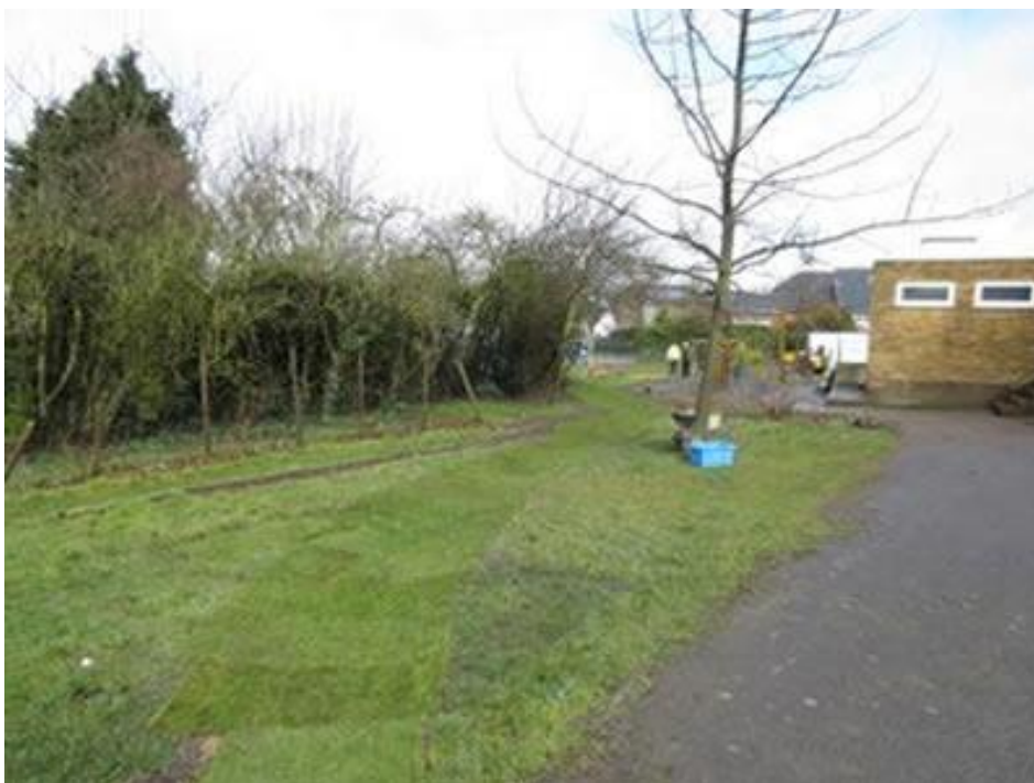
Figure 3 New tributary grass swale taking run-off from upper playground
