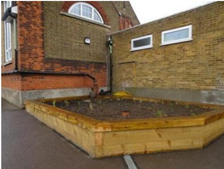
Figure 2 Bio-retention bog garden with seating showing disconnected downpipes and overflow drain
