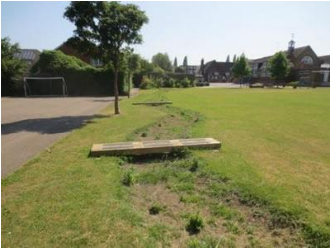
Figure 4 Detention area with bridges and planted with native plants
